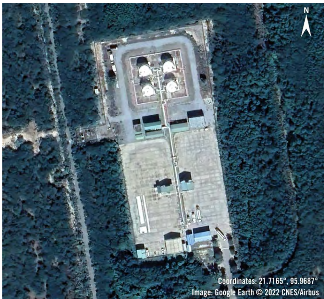
NEPAS storage facility at Mandalay airport.
