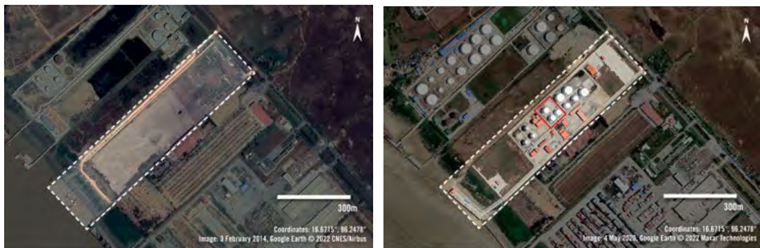
Puma Energy Terminal, Thilawa, Myanmar: Satellite imagery shows the Puma Energy Terminal while it was under construction at Thilawa (2014) and later in 2020, when the terminal appears to be operational. According to a company video, the three tanks used for jet fuel storage are shown in the image – highlighted with a red square.
