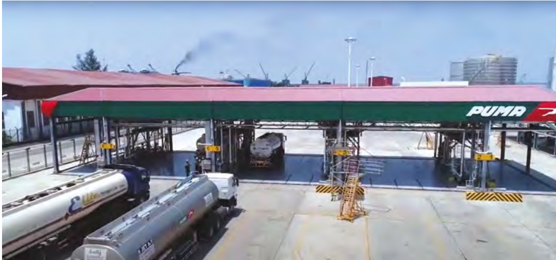
PEAS terminal, Thilawa port: The PEAS terminal has a loading bay where tanker trucks are loaded with the aviation fuel that is distributed to storage facilities across the country. 350
