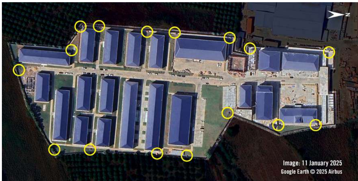
PSP01: compound with suspected guard posts - highlighted with yellow circles - at strategic locations within the perimeter wall.
