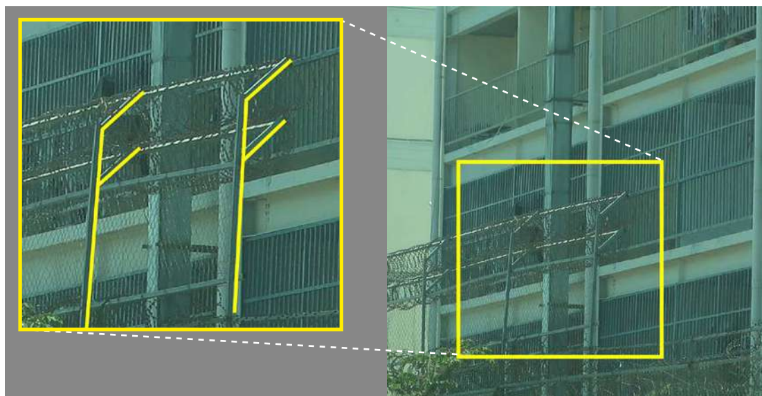
PP13: eastern perimeter wall is heightened and angled towards the interior with barbed or razor wire on the inside to prevent climbing. © Amnesty International, 2024.
