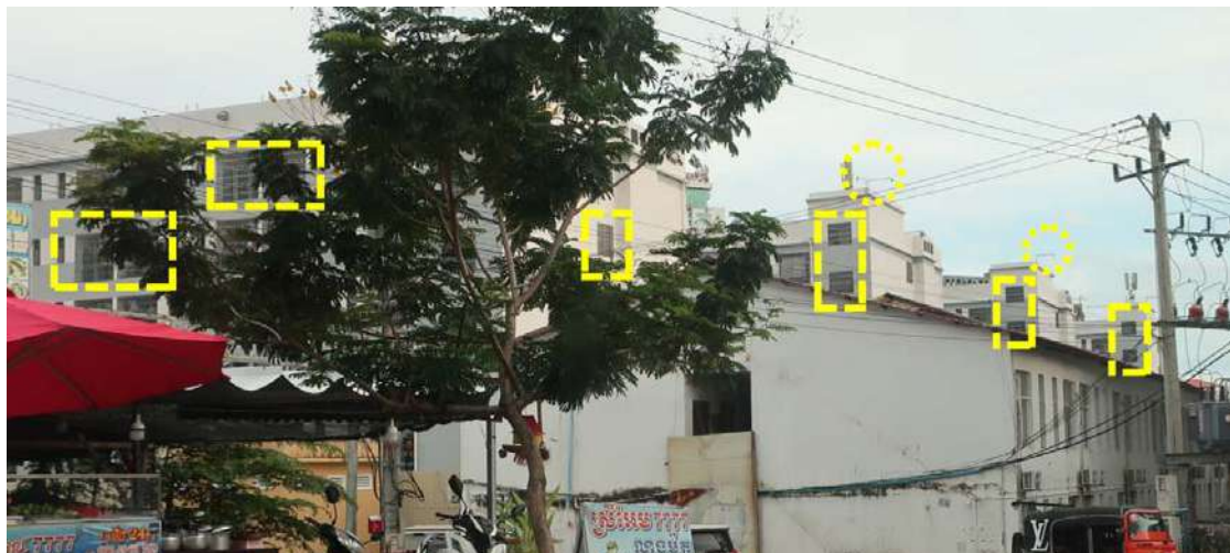
S108: security cameras can be seen on the roofs, and bars on the balconies and windows. © Amnesty International, 2024.
