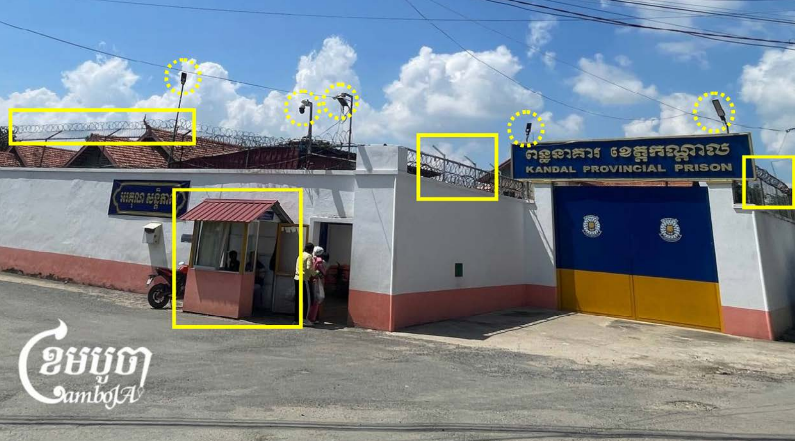
Kandal Provincial Prison; a typical Cambodian prison. Note the presence of a security guard or police officer; the use of barbed or razor wire that is angled inwards (internally facing) to prevent or make it more difficult to climb the wall from the inside; the use of walls that are too high for an average person to easily climb; the presence of security cameras, especially cameras that are internally facing; and the use of lights on the perimeter of the prison. Image from © Camboja News.
