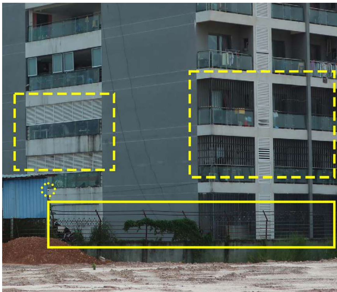
SI42: a guard tower positioned on the north-east corner facing inwards and along the northern wall of the compound. © Amnesty International, 2024.
