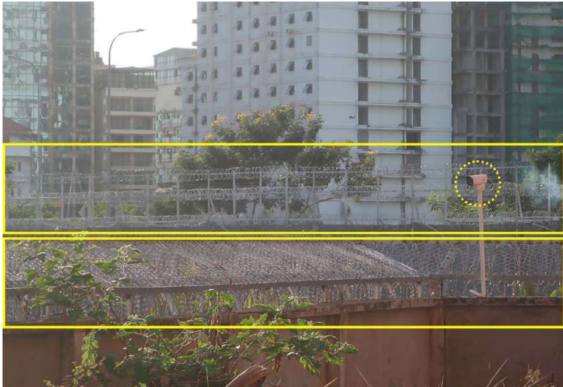
SI08, with its internally focused security cameras and razor wire that curves back into the compound, which local workers who constructed the fence described as looking “worse than a prison”. © Amnesty International, 2024.
