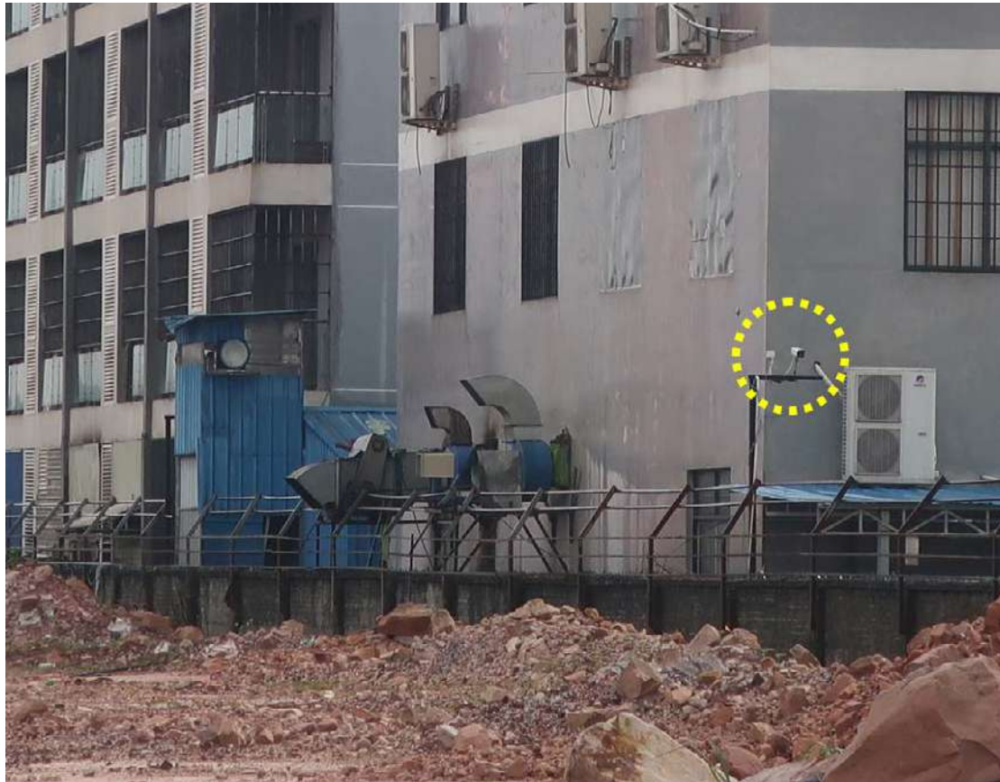
SI42: cameras in position to capture the northern perimeter wall. Note that the cameras are internally focused and appear aimed at filming the inside of the perimeter wall, rather than the exterior side. © Amnesty International, 2024.
